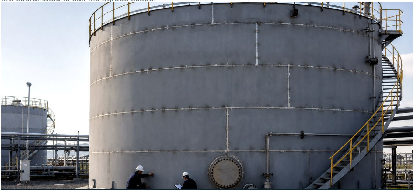
API 650 tank construction and field quality control
